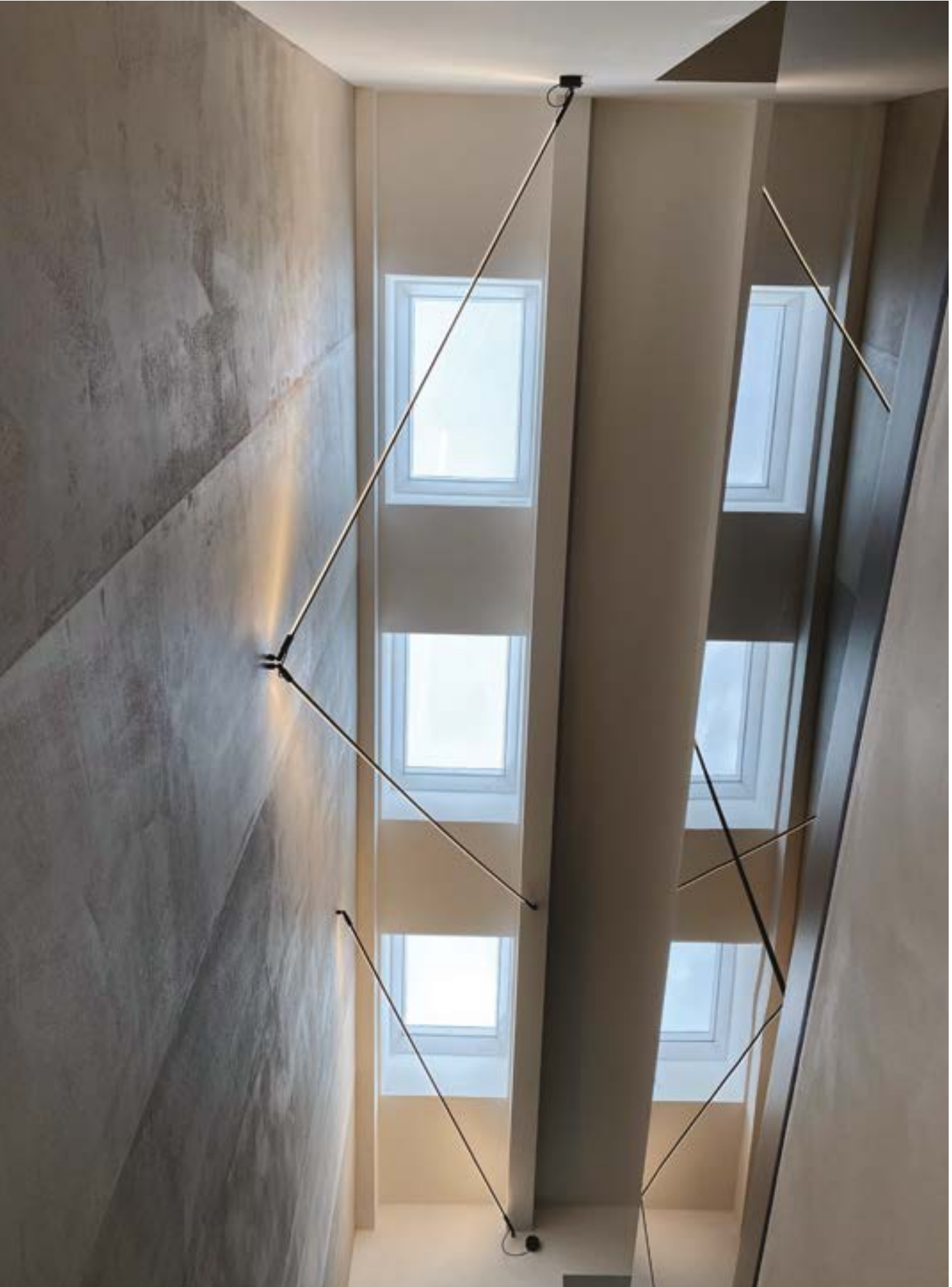
Installazione speciale con driver remoto e collegamento passante tra due profili Special installation with remote driver and pass-through connection between two profiles
